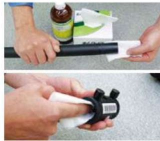
Cleaning the scraped surface and inner surface of fitting
