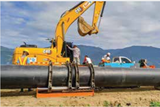
Instalasi Perpipaan SPAM PASIGALA, Sulawesi Tengah
